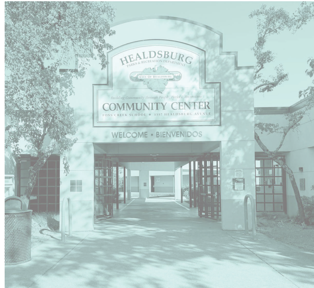
The entrance to the existing Community Center at 1557 Healdsburg Ave.
